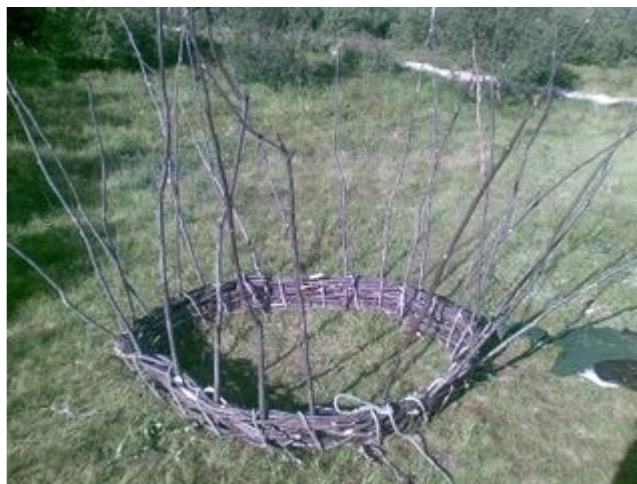
Figure 3: A rope was used to keep the weaving tight during construction
